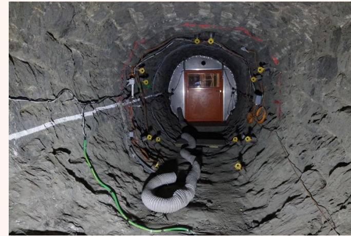
Closed niche ■ Controlled high humidity
