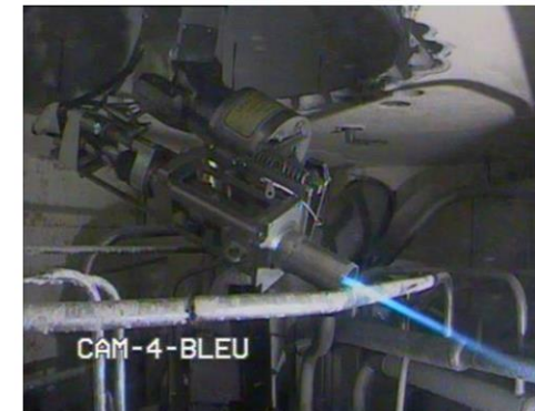
Up to 200mm in thickness in air (14kW laser power)
