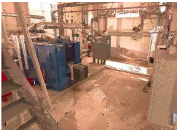
Figure 9: Point cloud of a boiler room (Daniska et al., 2021)
